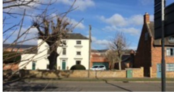
A visibly intrusive high roof line here behind much older buildings.
